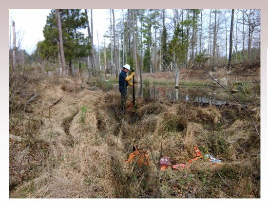
Before: Beaver had dammed the pond's overflow spillway causing a breach, which weakened the integrity of the pond dam structure.
