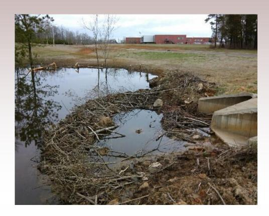
Before: A dammed culvert raised concerns for potential flooding at the entrance road to Granville County Central High School near Stem. It was also flooding an adjacent landowner's timber. Photo credit: Todd Menke, USDA Wildlife Services.
