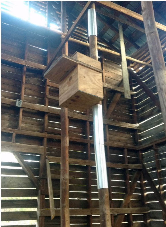
Flashing is used to deter predators from getting into the nest boxes. This one is posted in an old barn on Sandy Mush Game Land (Photo: Allison Medford)
