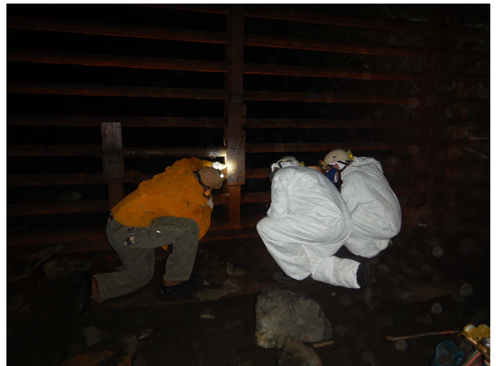
Conservation Technician, Joe Tomcho, Western Wildlife Diversity Supervisor, Kendrick Weeks, and Wildlife Diversity Technician, Kyle Shute, repair the bat gate inside an Avery County mine. (Katherine Etchison)
