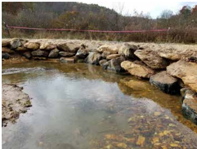
Figure 2. Large boulders and matting were used to stabilize the formerly eroding stream bank. The bog edge is immediately behind the pink flagging. Large gravel was laid down adjacent to the boulders to ensure the farmer could access his hayfield again. (Photo: Gabrielle Graeter/NCWRC)
